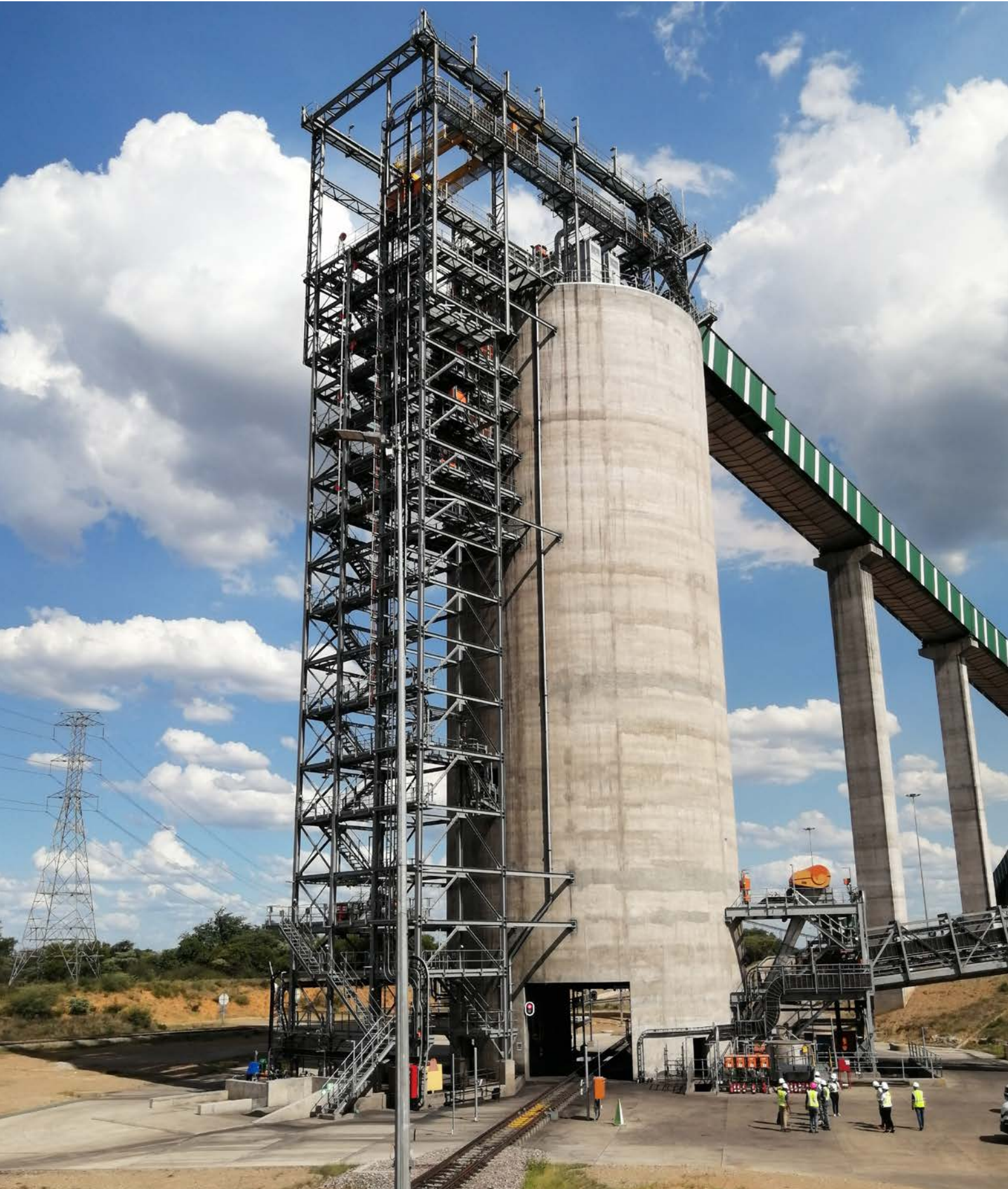
Load-out station at Grootegeluk
