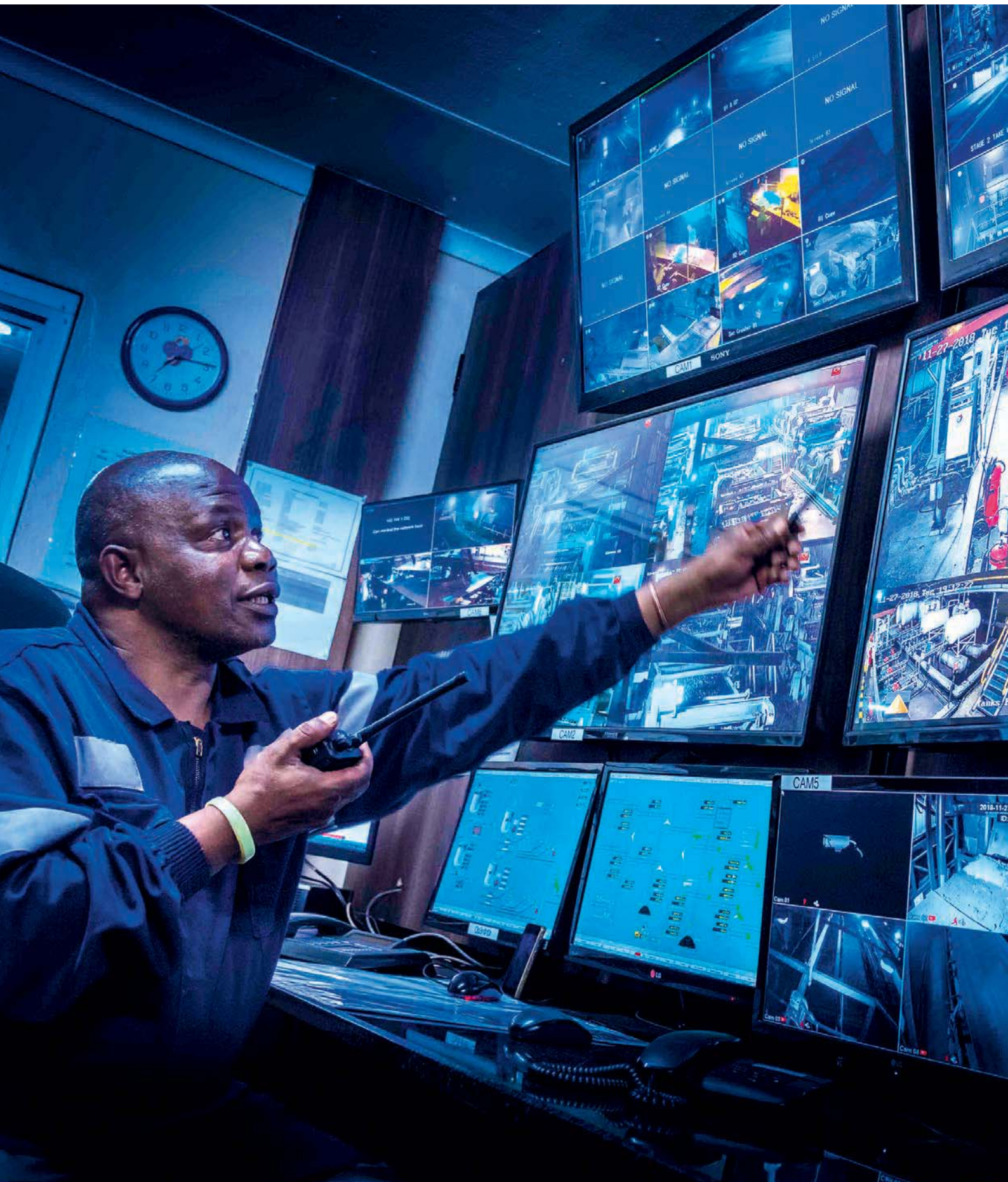
Digital operation centre at Matla
