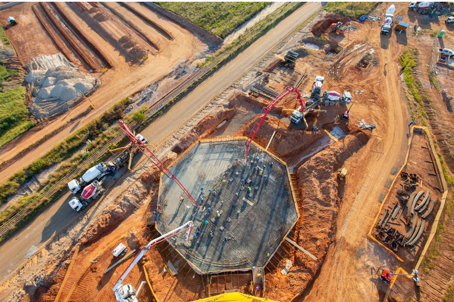
New shaft under construction at Matla Mine 1
