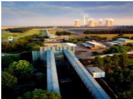
Figure 15: Matla conveyor system to the power station
