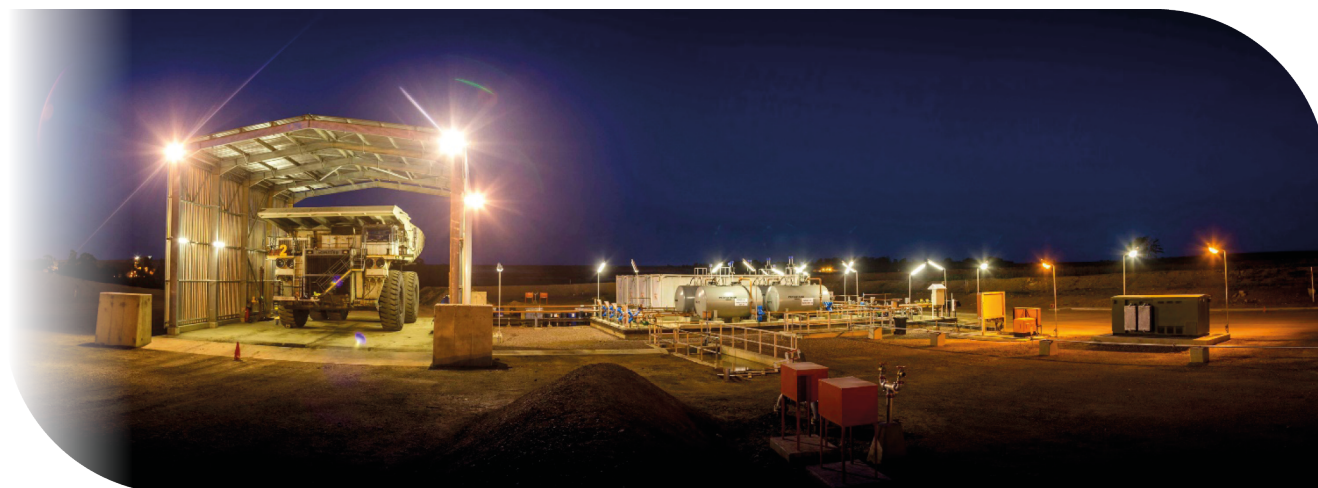
Service bay for production trucks
