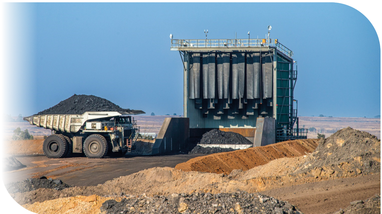
Offloading coal at the tip bin at our Mafube open-pit operation, Mpumalanga
