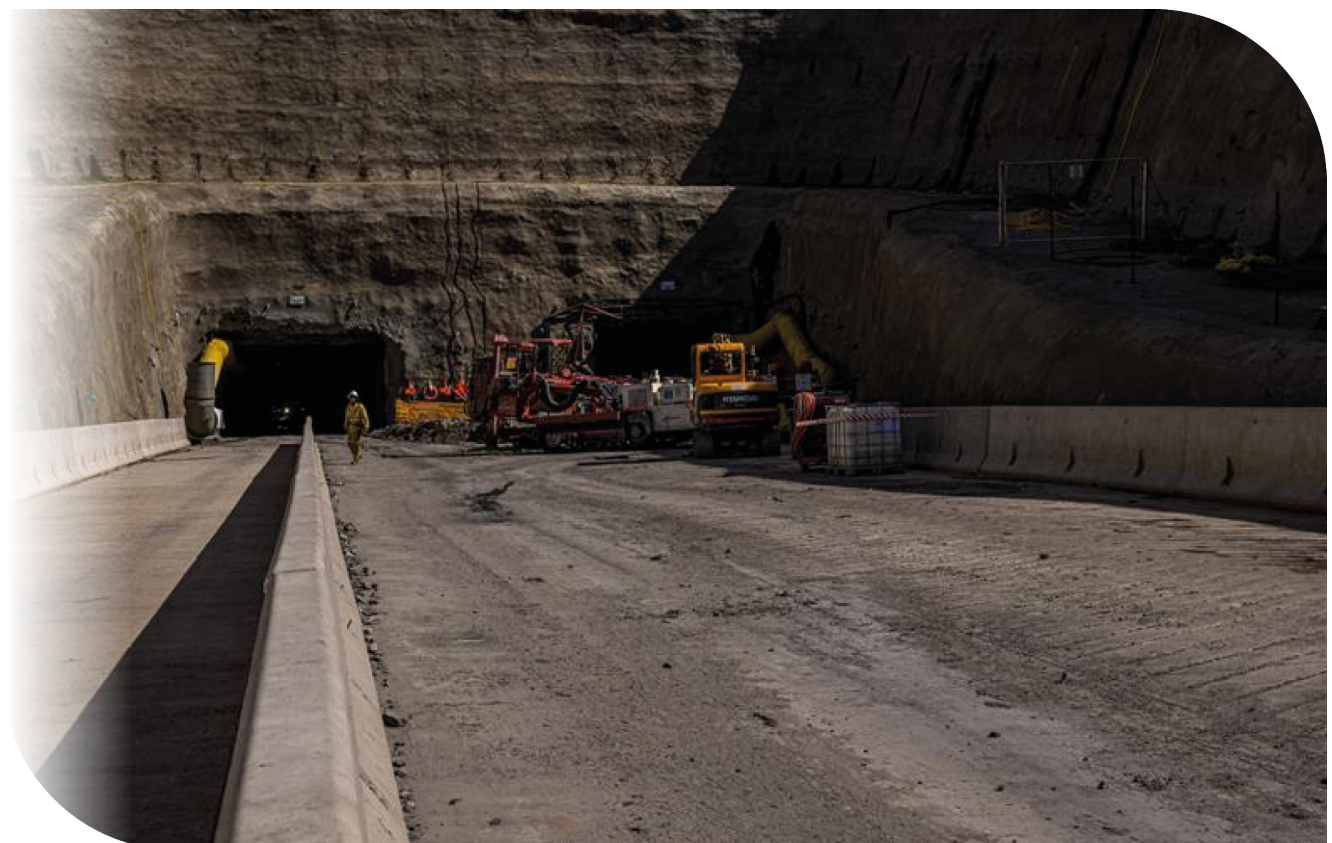
The new entrance to Matla Mine 1
