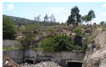
Successful sealing of adits at Hlobane mine
